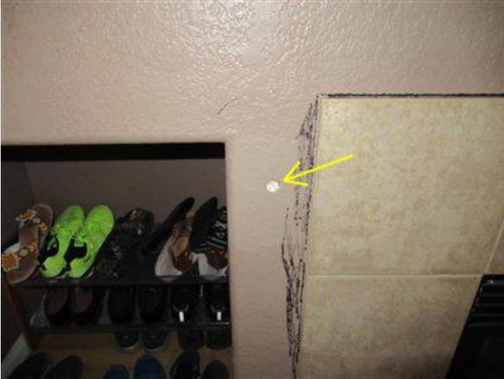
Photo 27-1 Next to fireplace
