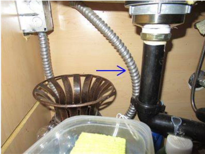
Photo 5-1 Below kitchen sink
